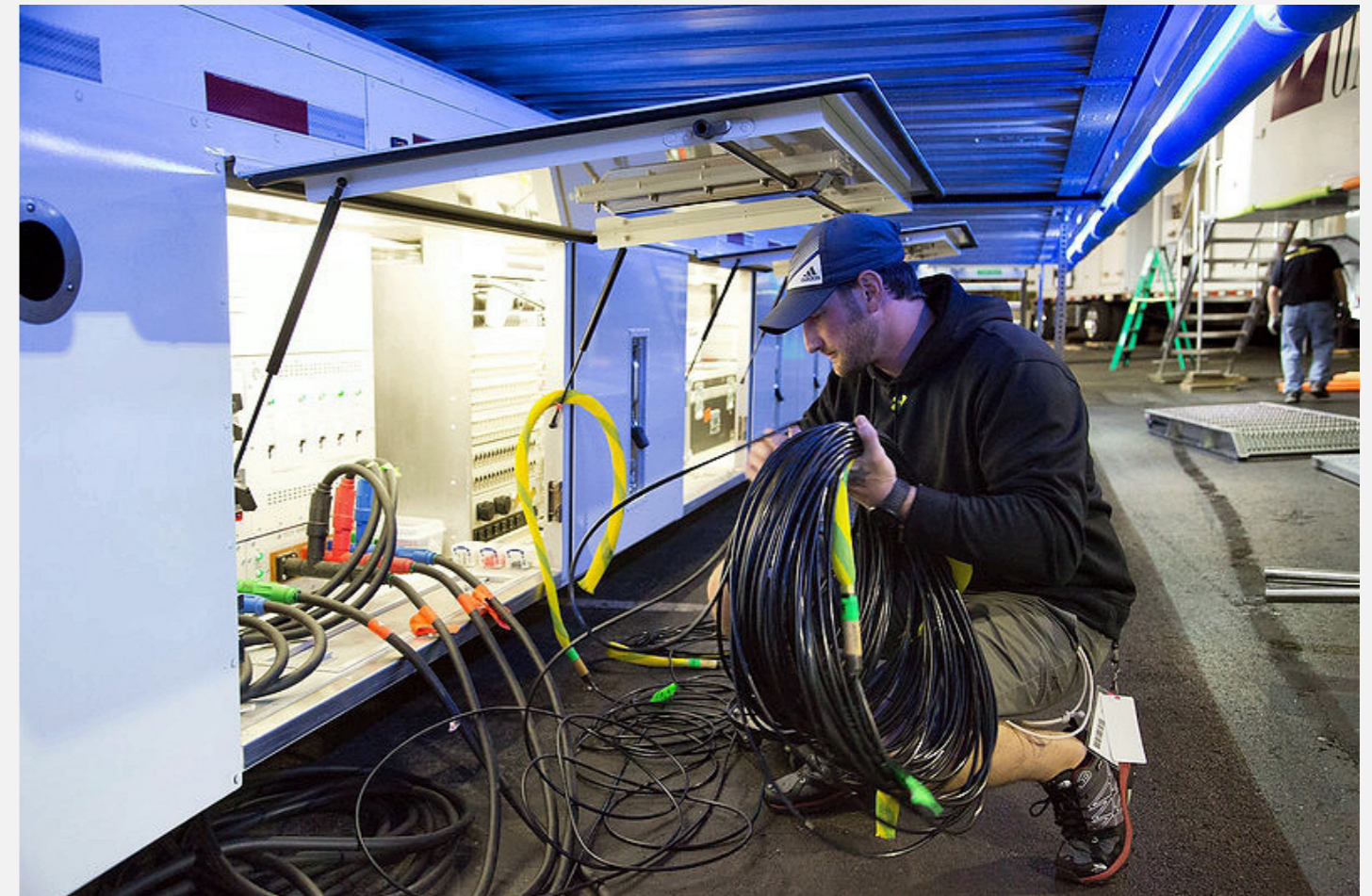
Technician pulling fiber.
